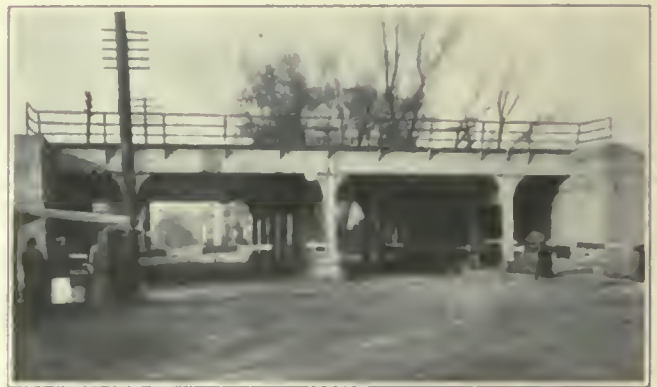
FIG. 279. TRACK ELEVATION. Deck plate-girder bridge of the Chicago & North Western Railway at Harlem Avenue, Oak Park.
